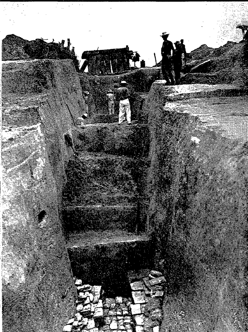
DEEP TRENCH exposing buried pavement offering. The columned tomb appears at the top.
